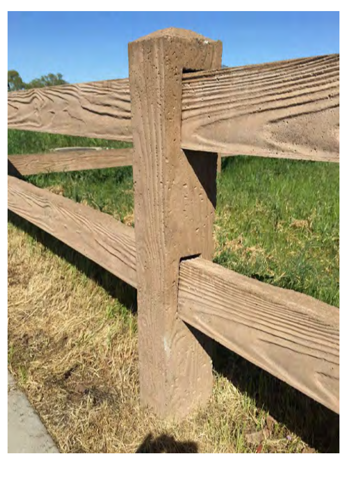
PRECAST TWO-RAIL FENCING: COLOR: 'EARTHTONE BROWN', AS MANUFACTURED BY DYNAMIC PRECAST, PHOENIX PRECAST, ARTISAN PRECAST, OR EQUAL, INTENT: NATURALISTIC COLOR, FENCING TO VISUALLY RECEDE (PER HPCO DESIGN GUIDELINES)
